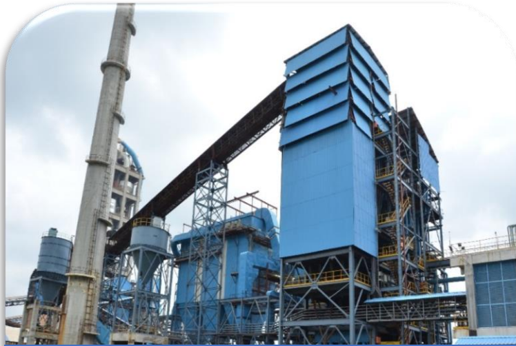
THERMAL POWER PLANT, MUKTYALA – 1X18 MW
