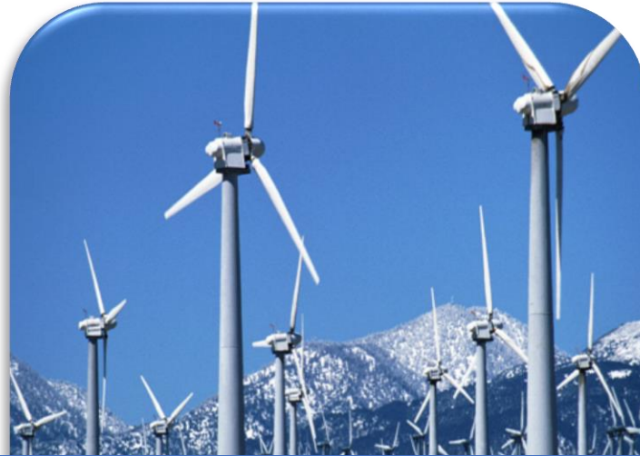
WIND POWER, THIRUNELVELI – 3.25 MW
